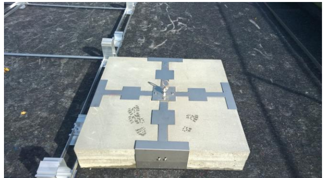
Fig. 4: Stonekit load system with rope system from Grün GmbH ( www.gruen-gmbh.de ) in combination with MSP-FR-EW.
