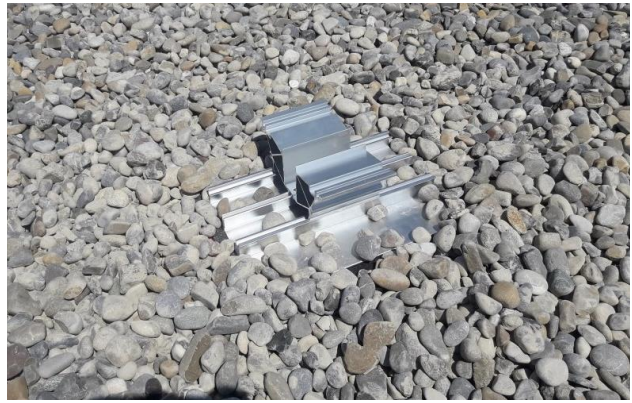
Figure 6: Shallow covering of the intermediate layer with gravel
