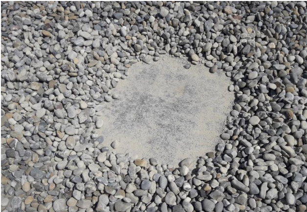
Figure 3: Clear local area of gravel completely
