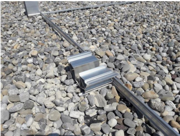
Figure 7: Support with mounted connecting rail
