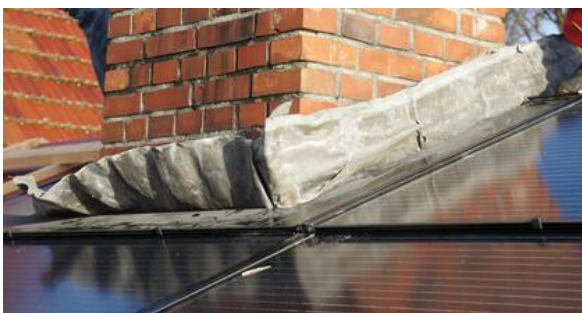
Abb. 3: Anschlüsse an Kamin
