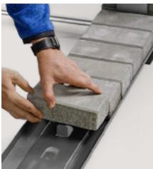
For exposed locations, ballast fixation guarantees maximum safety, with ballast blocks in longitudinal and transverse direction. Laying is achieved without tools. Thanks to the flexibly positionable and pre-punched tabs, ballast blocks can be fixed precisely and without gaps, perfectly in line with the calculated ballast volume.
