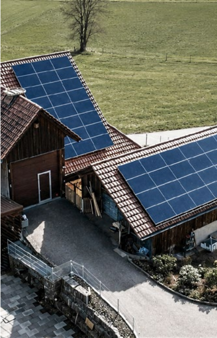
MSP-PR on-roof inlay Cham (Switzerland)
