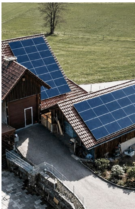
MSP-PR on-roof inlay Cham (Suisse)
