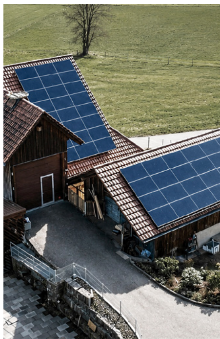
MSP-PR on-roof inlay Cham (Suisse)
